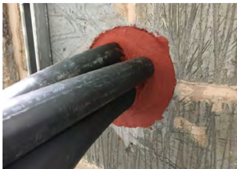
Fire seals around cables and trunking.
