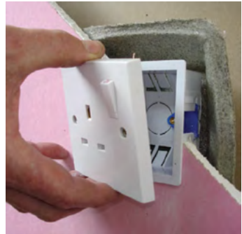
Fire and acoustic rated covers fitted behind dry lining box (Photo courtesy of Tenmat Ltd).
