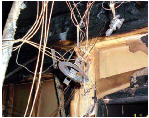
Result of a downlighter fire (Courtesy of Manchester City Council - Building Control).
