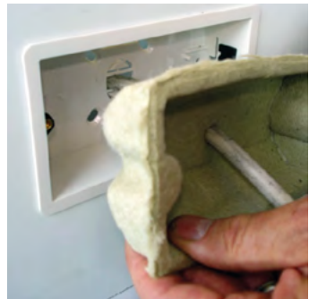
Intumescent pad being installed in a dry lining box (Photo courtesy of Knauf Drywall).
