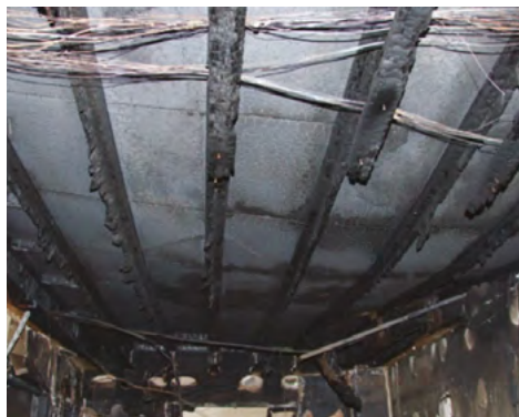
Result of an eight minute fire on lightweight joists (Courtesy of Manchester City Council - Building Control).
