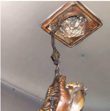
Fire spread into bathroom via plastic duct (Photo courtesy of Greater Manchester Fire & Rescue Service).
