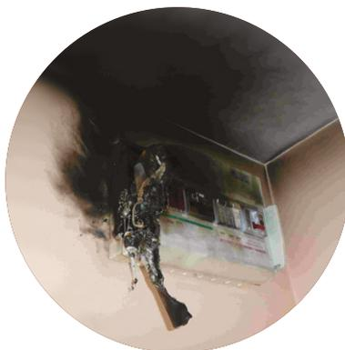
*Result of DIY work by a home owner where a 10.5 kW electric shower was connected to a 45 A circuit-breaker using 2.5 mm<sup>2</sup> cable. (Photo courtesy of British Gas)*
