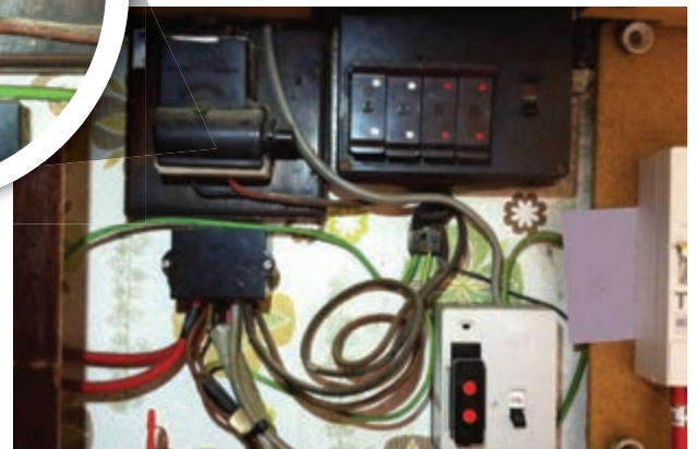
Right: Relatively modern meter fitted to potentially dangerous installation.
