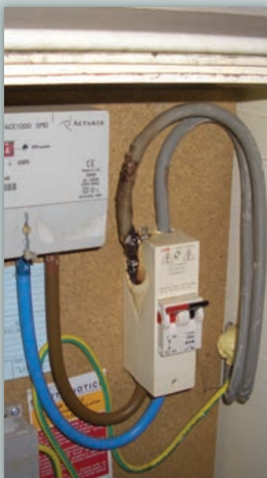
Electrical intake fires are caused by resistive heating at loose or deteriorating connections.
