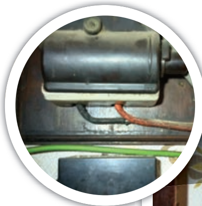
Top: Perished vulcanised rubber insulation adjacent to meter.
