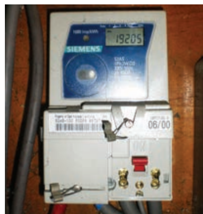
Existing meter with integral isolating switch (cover removed).
