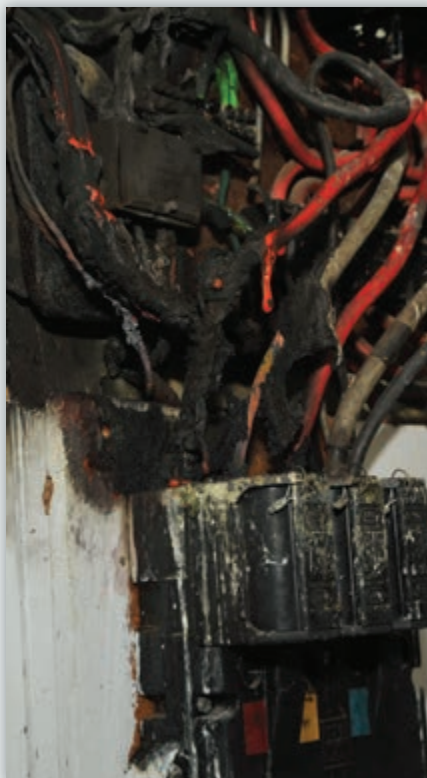
Consequences of overheating cut-out fuse assemblies.
