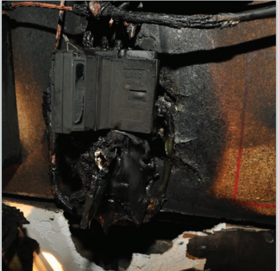
Consequences of overheating cut-out fuse assemblies.
