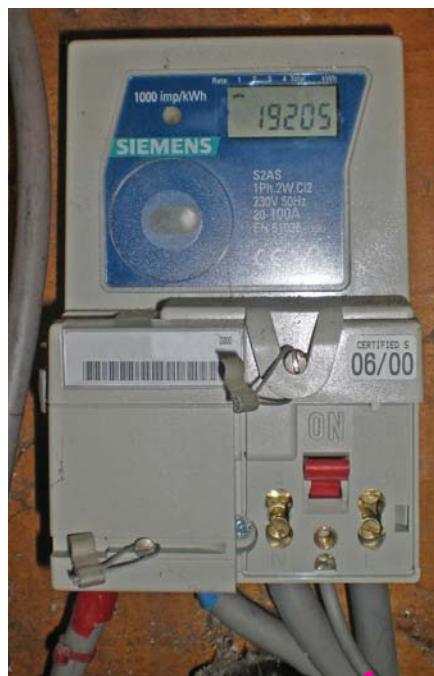
Existing meter with integral isolating switch
