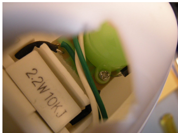
Figure 4 View of accessible live parts
