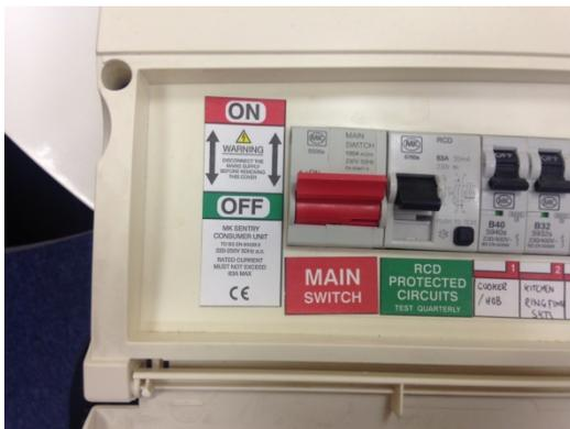
Sometimes it will be necessary to operate more than one switch in order to isolate a single source of supply to all parts of the property (more than one consumer unit) or because the installation is fed from a distributed mains supply and also an alternative supply from, for example, a solar photovoltaic (PV) system.
