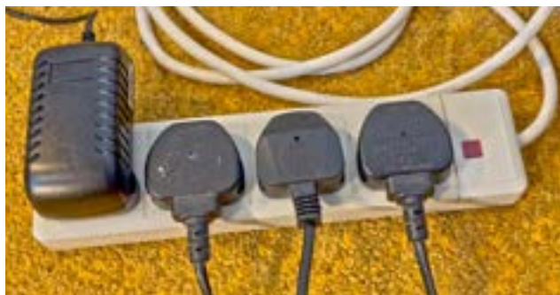
Figure 02: Example of a multiplug extension lead.
