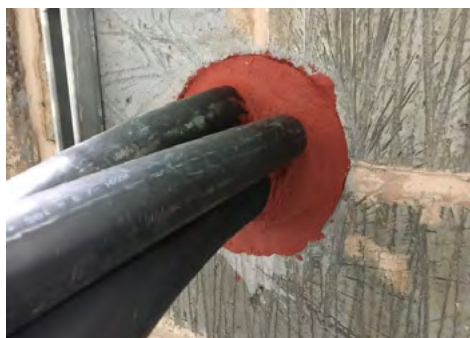
Fire seals around cables and trunking.
