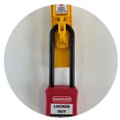
Where lockable inserts are not available, care should be taken to ensure that no 'spare' fuses or fuse carriers are left in the proximity of the distribution board. A prohibition sign should be attached at the point of isolation to deter others replacing the fuse with a spare and energising the circuit, and the following must be considered:
