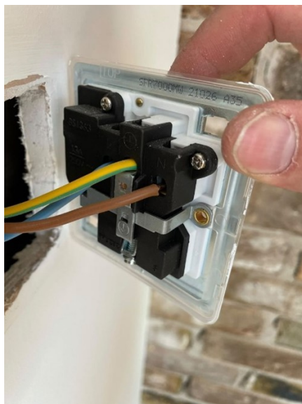
Inspecting a socket-outlet
