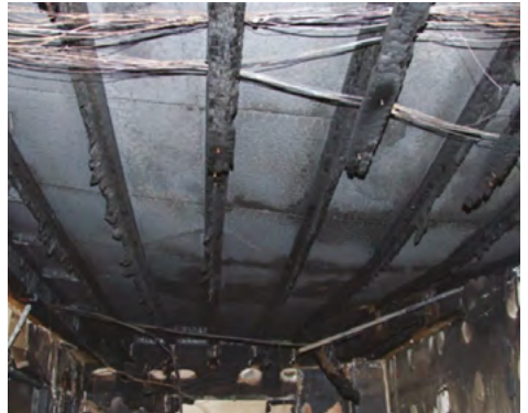
Result of an eight minute fire on lightweight joists (Courtesy of Manchester City Council - Building Control).
