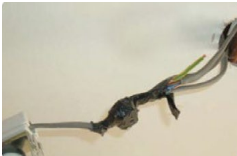
Unsatisfactory connections to a downlighter, requiring a Code C2.
