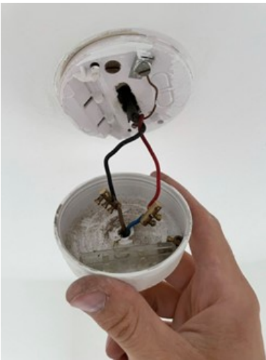
Inspecting a ceiling-rose
