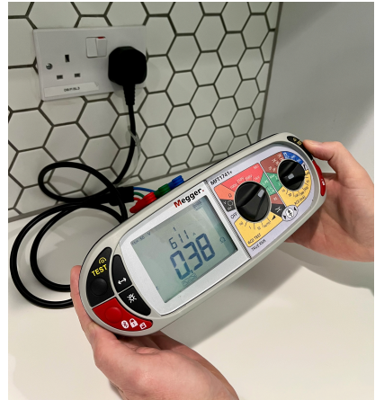
Electrical tests being carried out.
